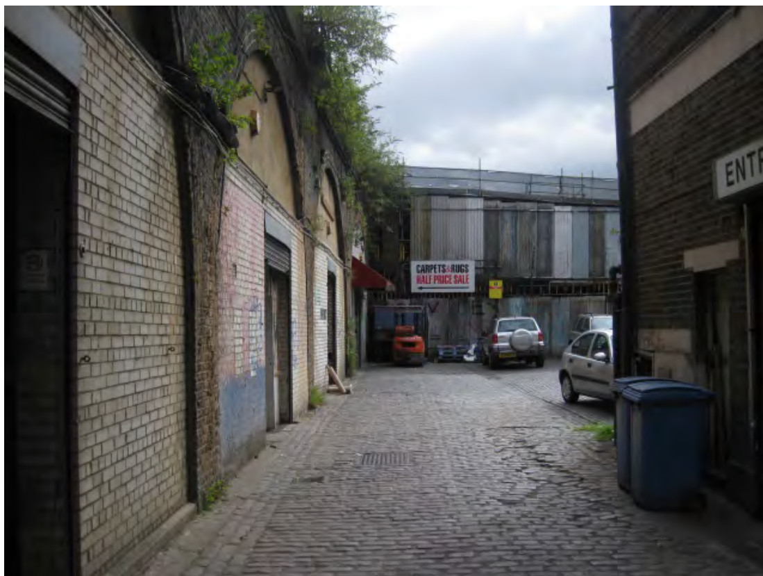
PNAAP 3: Land between the railway arches (East of Rye Lane including railway arches)
